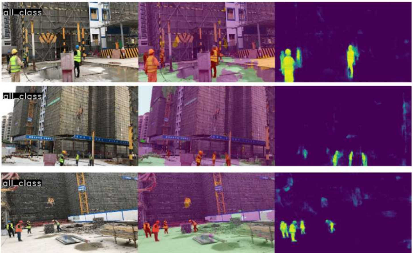
Figure 3.3.1: The original image can be seen in the image on the left. The output of the detections superimposed on the original image is seen in the middle image. The confidence(output) in human segmentation at each pixel position is shown in the image.
