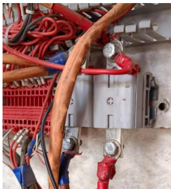
Fig.34. Mounting of bolted type terminal block
