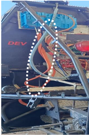
Fig.64. Motor controller, Motor HV wiring route inside a conduit
