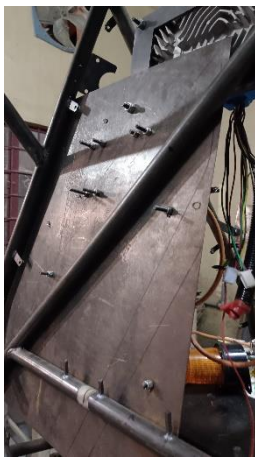
Fig.41. Mounting position and plate fixed during fabrication phase
