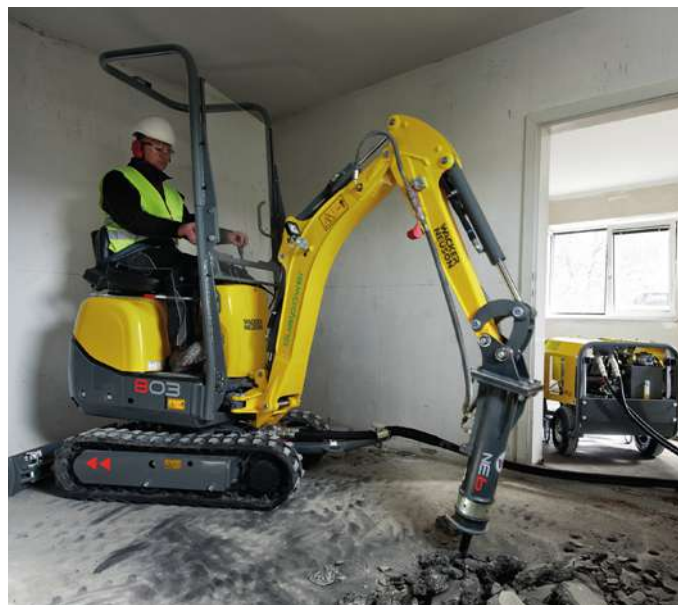
Operators of the 803 dual power excavator have a machine that offers the features of a conventional diesel excavator, but at the same time also could use the HPU8 generator emissions-free applications.
