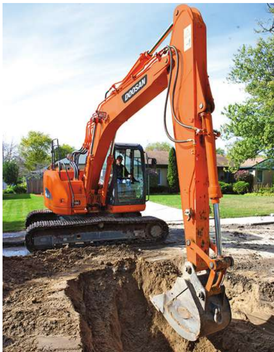
Doosan has added more power, performance, and speed to the 16-ton (14.5-t) excavator market with the T4 Interim DX140LCR-3, providing greater capabilities for site development.
