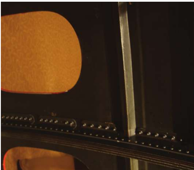
Close-up of a 787 fuselage panel showing the composite structure with metal fasteners and strengtheners. (Richard Gardner)
